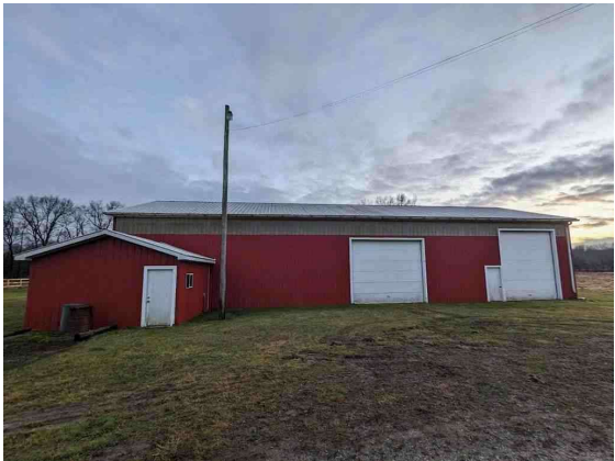
Machinery Shed Exterior
