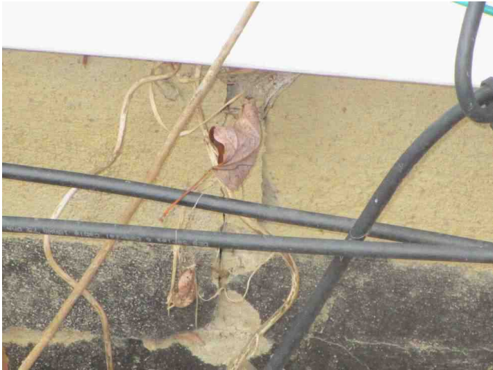
Foundation (settlement detail)
