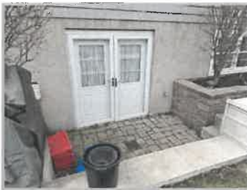
Outside Entry from Basement
