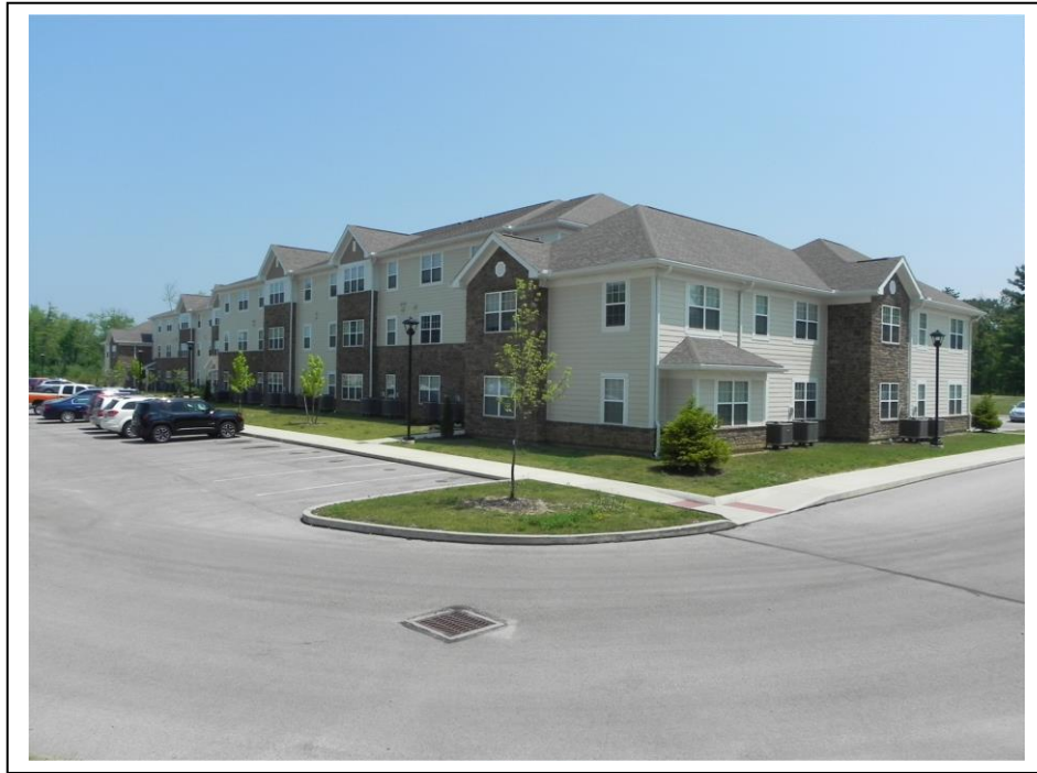
Front View of Improvements
