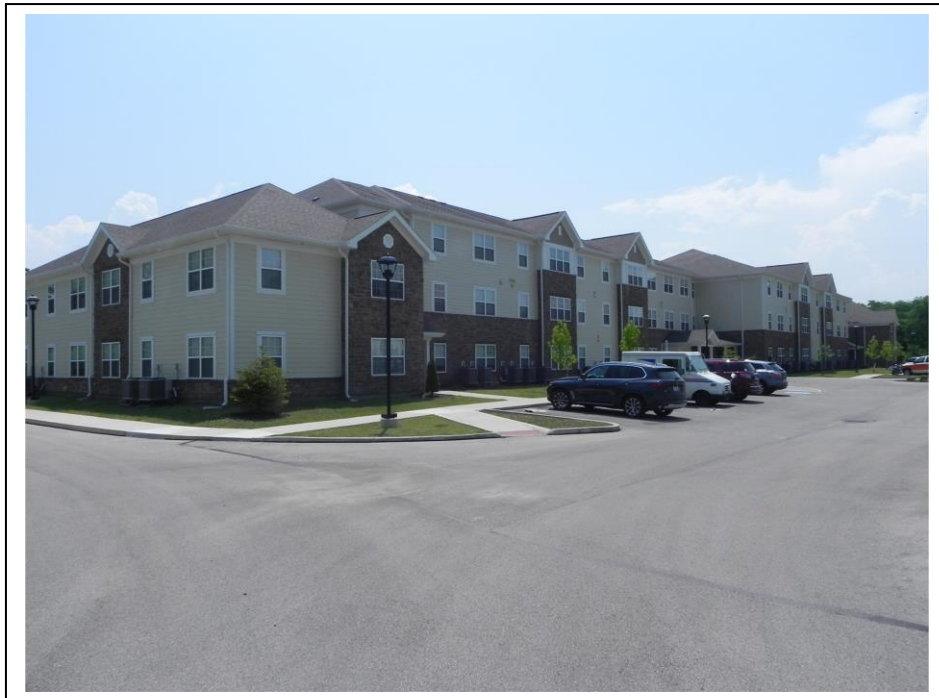
Front View of Improvements
