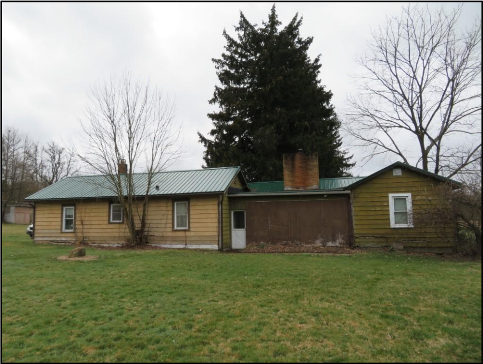
REAR VIEW OF SUBJECT PROPERTY
