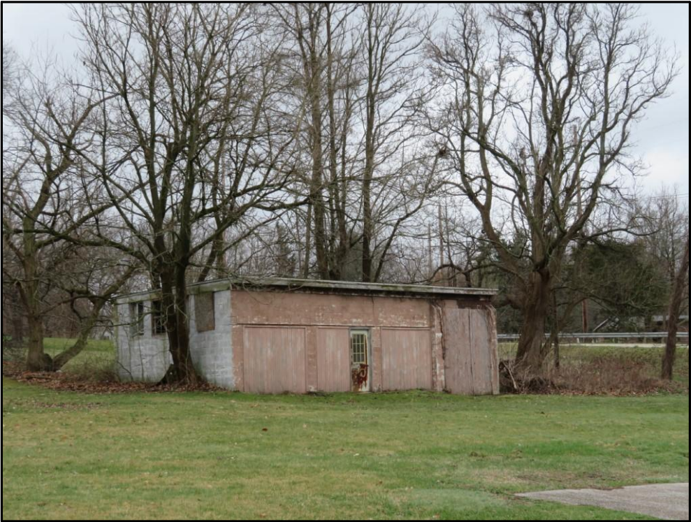
East and north sides of outbuilding
