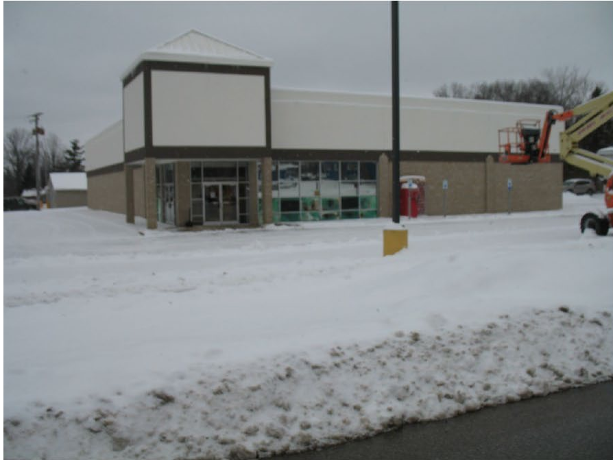
Figure 1 Subject front elevation and main entrance
