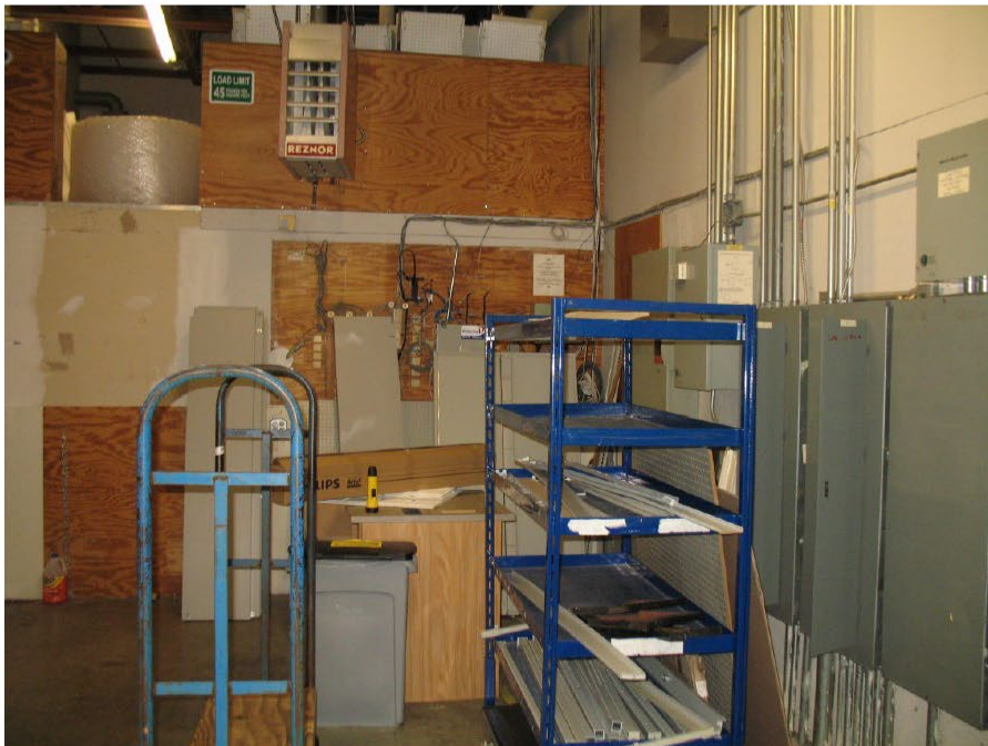
Figure 8 Storage area at rear of building
