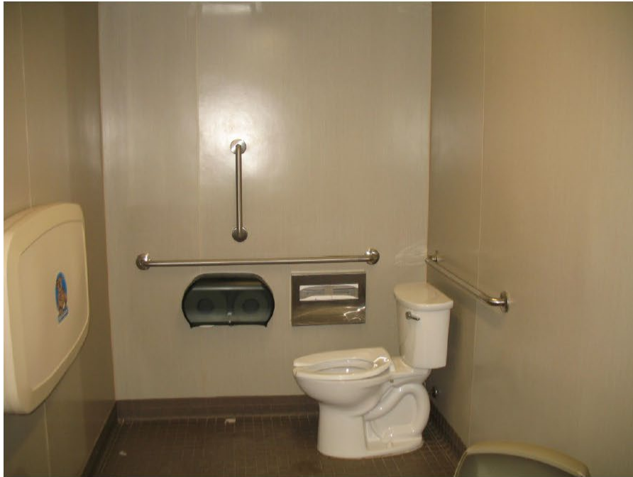
Figure 9 Restroom in rear storage area
