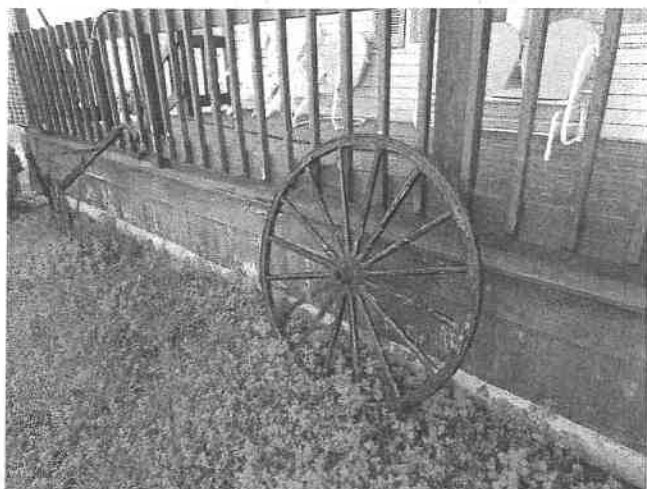
PEELING PAINT (Front Porch)
