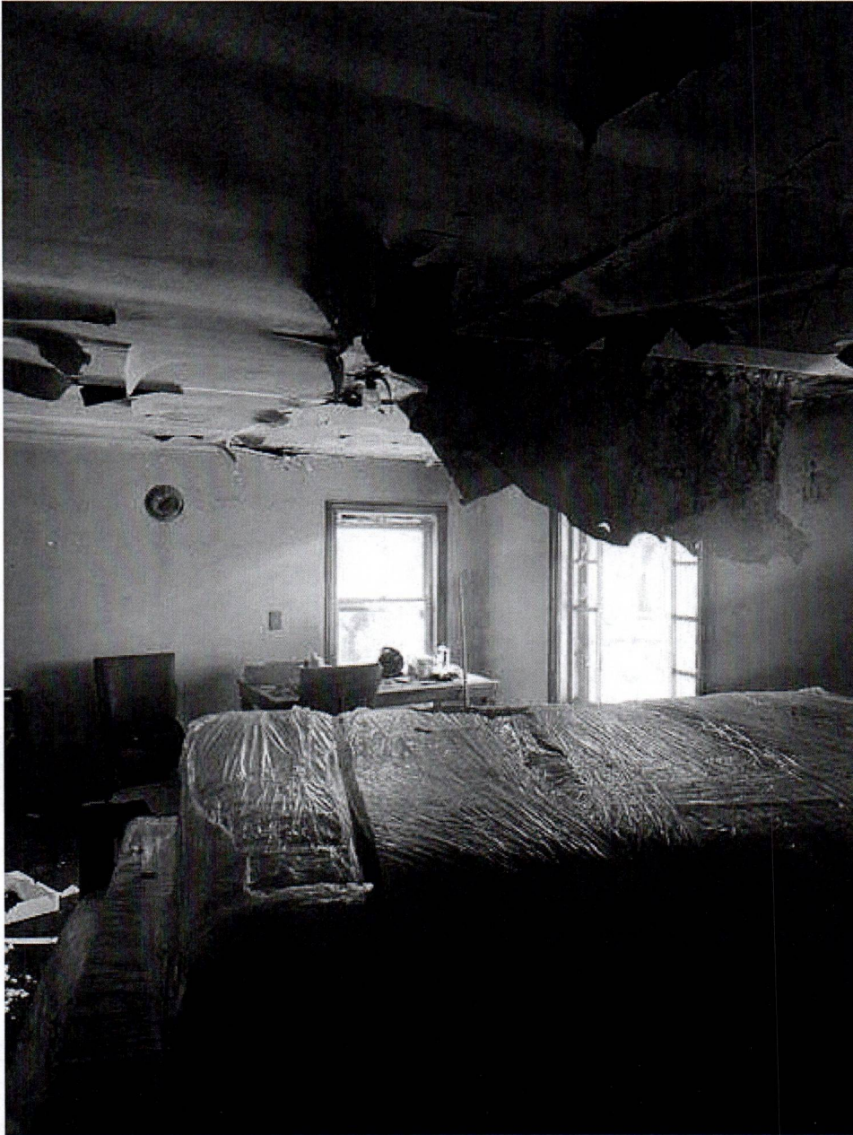
ceiling in one bedroom
