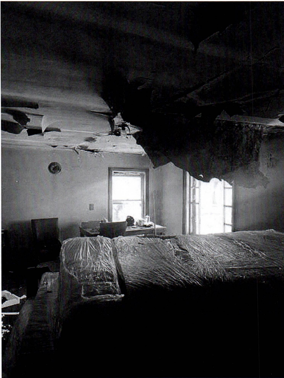
ceiling in one bedroom
