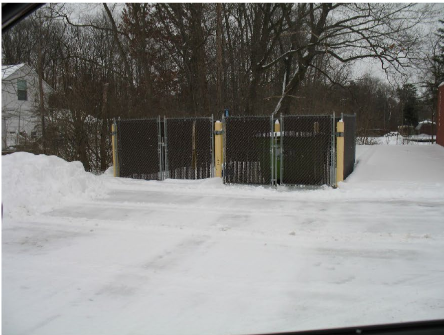
Figure 4 Dumpster and storage enclosure
