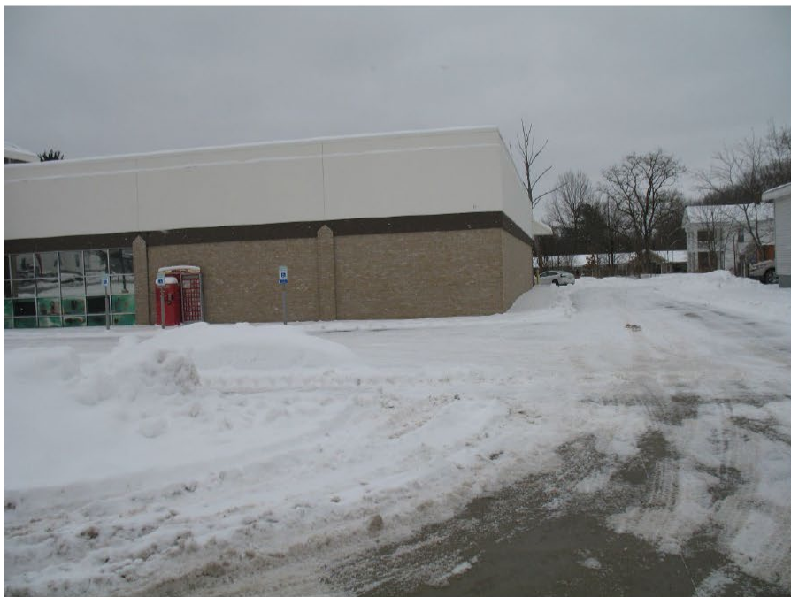
Figure 2 Rear Ashtabula entrance drive and rear of building
