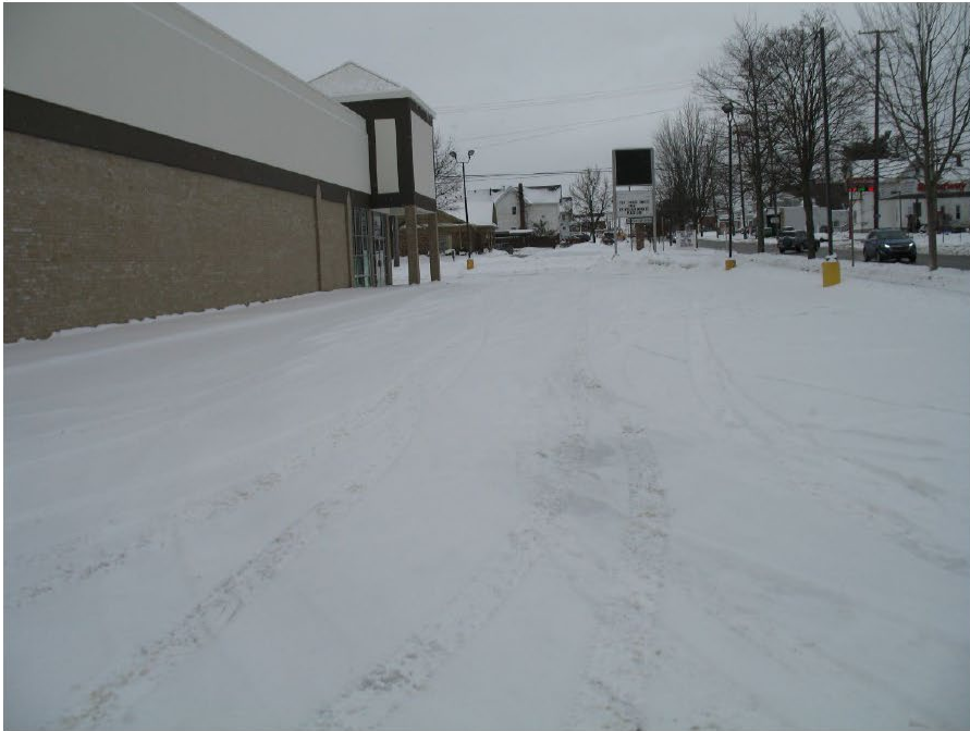
Figure 3 West building elevation and parking lot along N. Chestnut Street
