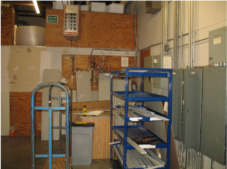
Figure 8 Storage area at rear of building
