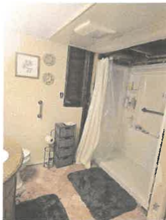
full bath photo 2 of 2 (ceiling of shower - unfinished)
