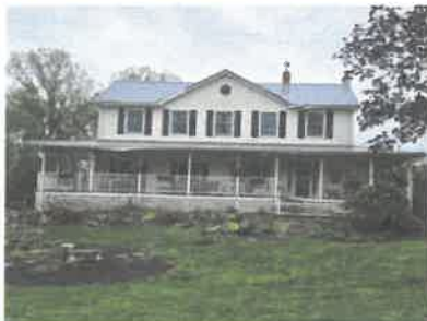
Farmhouse featuring a porch, a chimney, metal roof, and a front lawn
